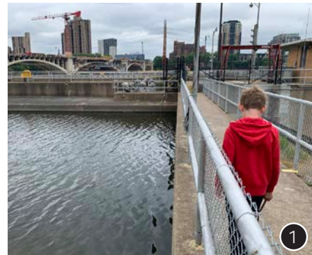
View: On the Lock, facing east to Stone Arch Bridge
