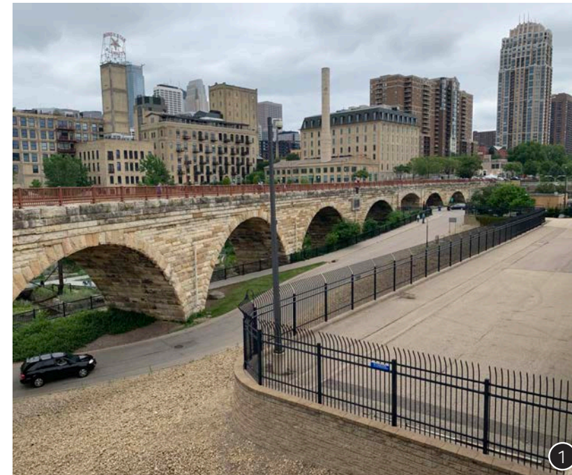
Stone Arch Bridge and fenced central control station platform on top of sand slope
