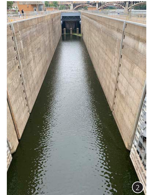
Decommissioned Lock and Dam
