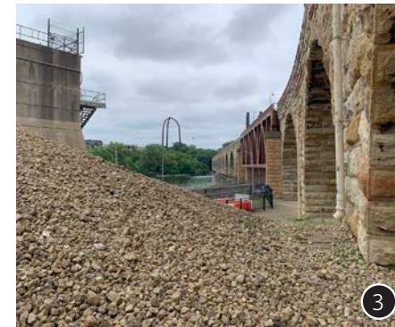
View: Under the Bridge, facing north
