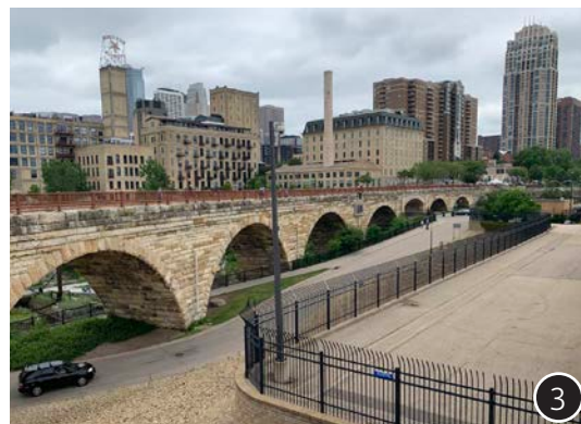
Stone Arch Bridge and fenced central control station
